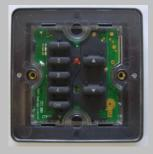
Unscrew and remove Front from Wall plate
